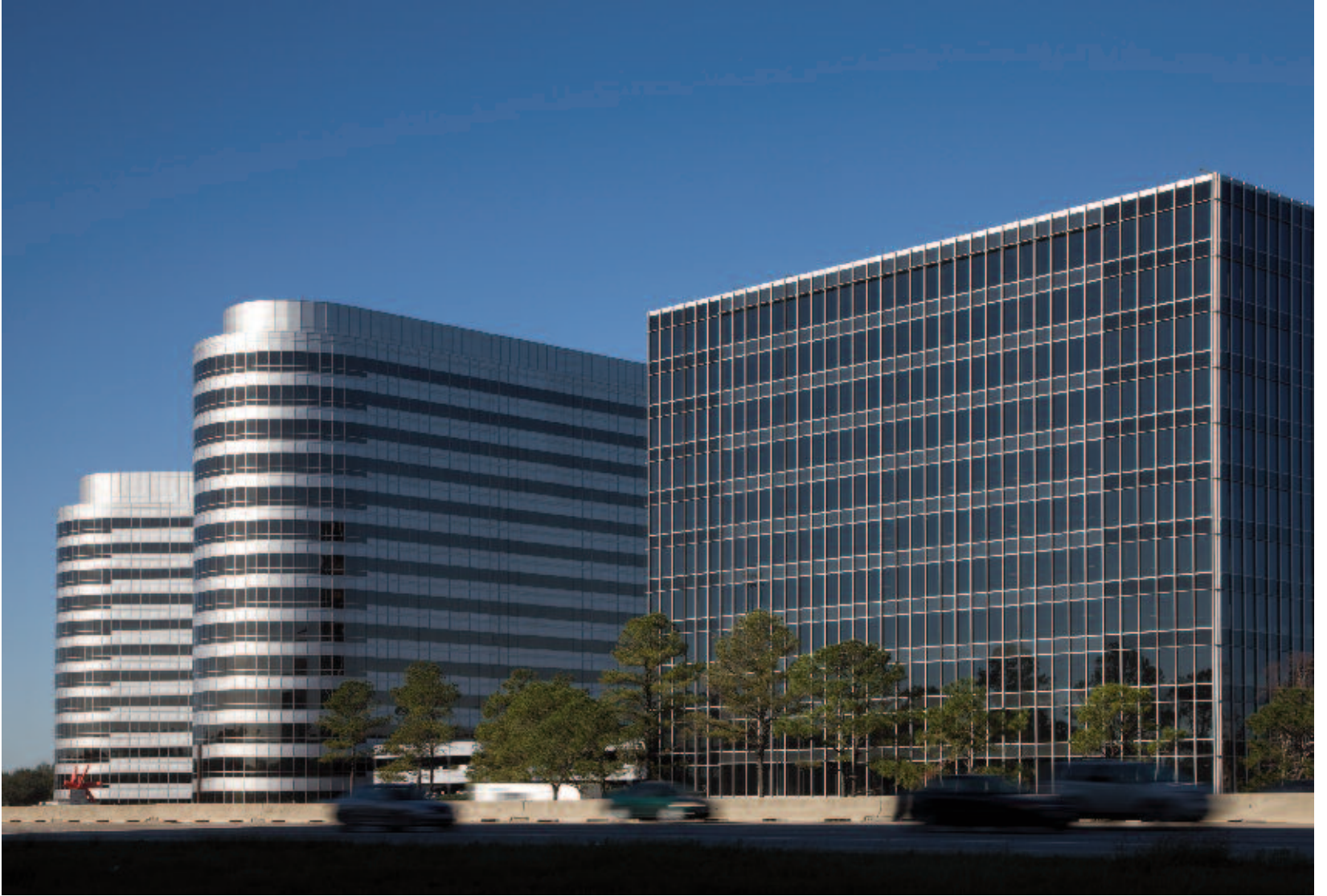
Brookhollow Central I-III, Houston, TX
